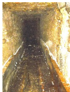
Installation of wooden panels
