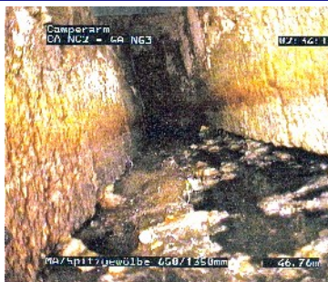
Almkanal before installing the Rabtherm System
