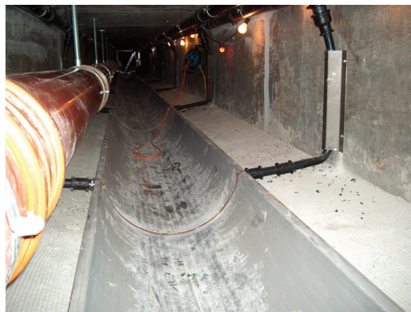
A sewer pipe equipped with the Rabtherm Energy System
